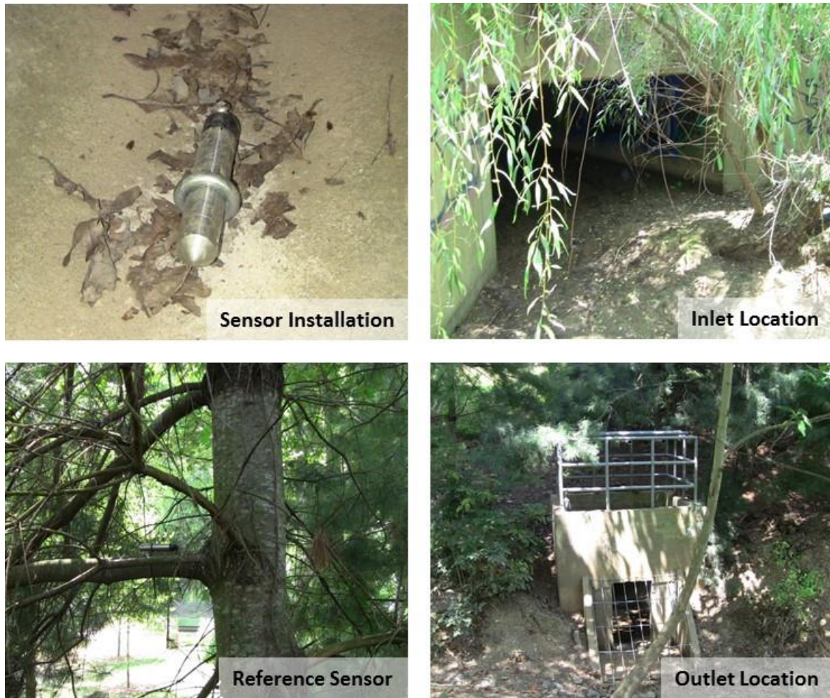
Figure 1. Installation of Hydrologic Monitoring Equipment in the Arboretum.
